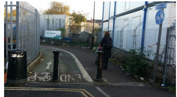
Poor quality pedestrian links in the area
